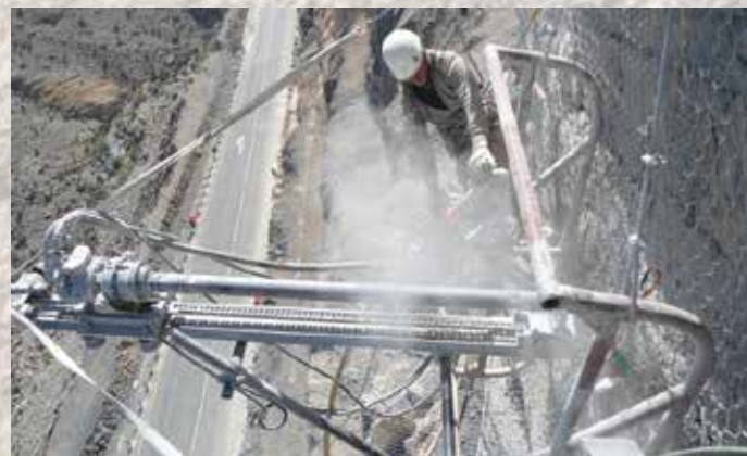
Drilling at high elevation with saddle and specialized climbers
