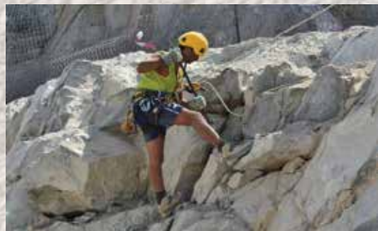
Scaling and removal boulder at high elevation with specialized climbers
