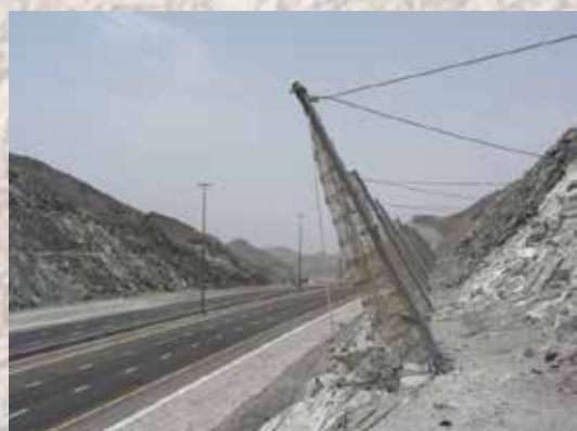
Drilling with rigs on basket
